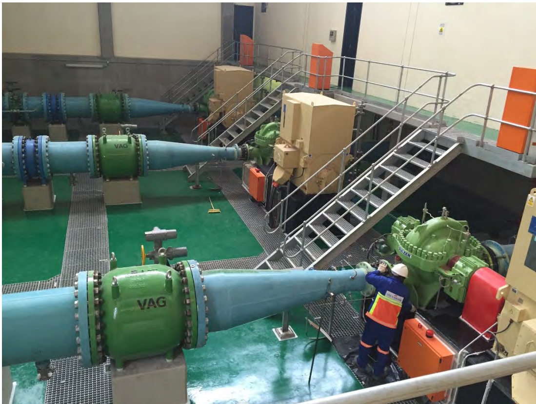
Mokolo High Lift Pump Station (109MI/Day at 245m head)
