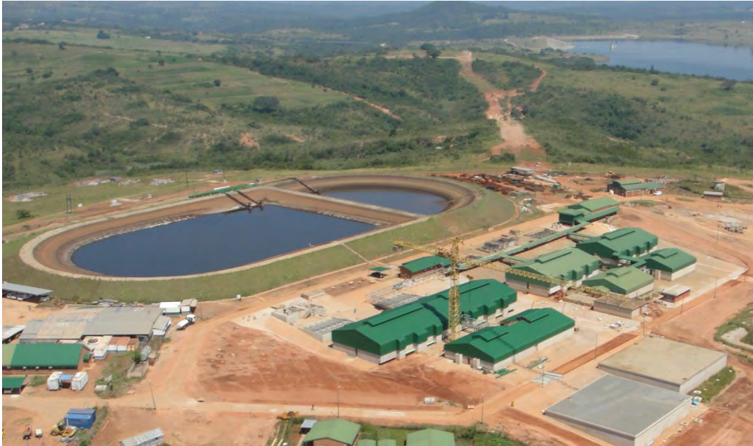
Inyaka Water Treatment Plant in construction phase (100MI/Day) - Aerial View
