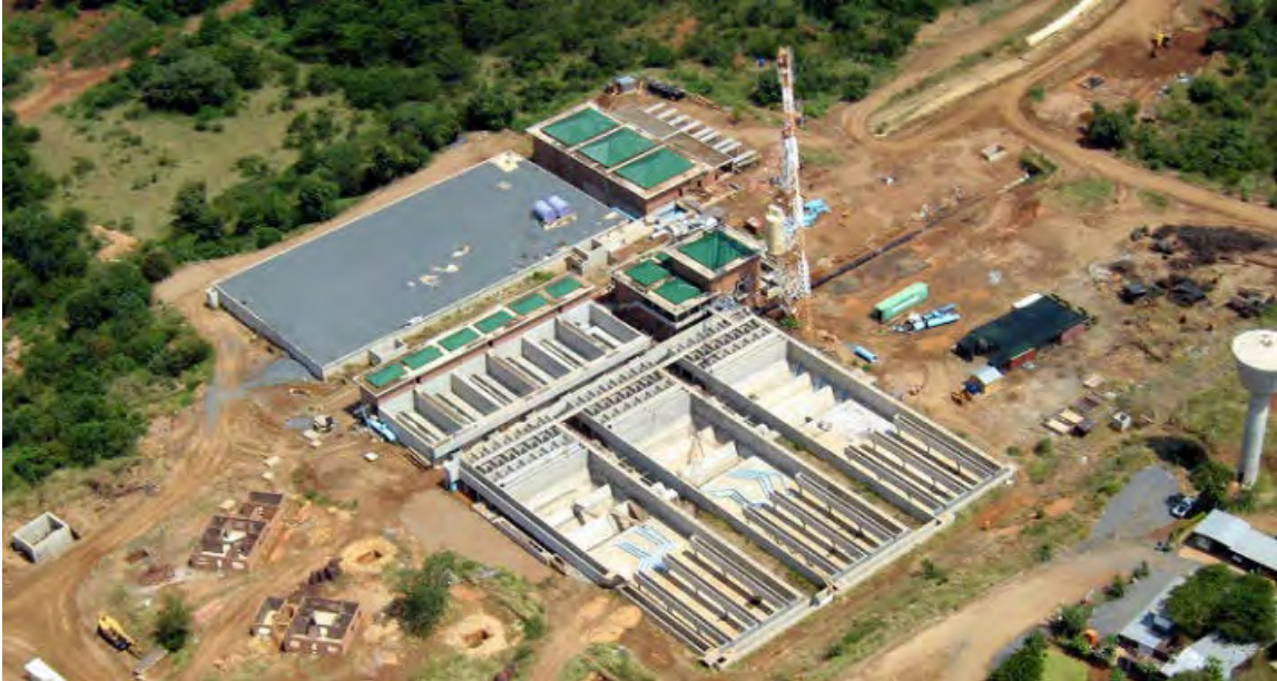
Nandoni Water Treatment Plant in construction phase, (60MI/Day) - Aerial View
